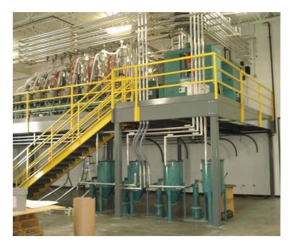
Air handling equipment for your facility, automated water treatment equipment for chemical processes, conveyors for materials handling and feed hoppers for automated equipment can all be easily moved to mezzanines. Easy access can be maintained to this equipment via the same mezzanine that supports it.
